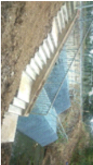
2. Mexborough Road, Adwick on Dearne - Trash Screen Checked before any predicted heavy rainfall events to assess requirement for cleansing.
