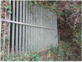
1. Bowland Close, Bentley - Trash Screen Checked before any predicted heavy rainfall events to assess requirement for cleaning.
